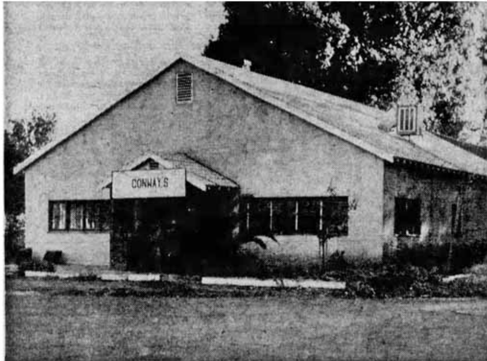
... Customers who have been getting their Indian herbs at Conway's Store will soon be buying them at a new location. Mrs. Juanita Simpson, who has operated the business at the Indian Village since 1954, is building a new structure at the corner of West Sacramento Avenue and North Cedar Street. The Conway family has been in the herb business for some 30 years ...
